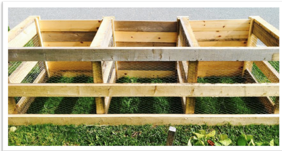
3-bin Composting System – Built in Summer 2014
